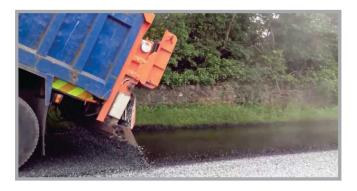
Mamz ChipSeal CRS2® consists of small bitumen droplets stabilized with chemicals that are dispersed in water allowing the bitumen to uniformly coat the aggregate even under cold conditions, Its strong hydrophilic properties displace the water from the aggregate, creating a strong bond with the stone during the breaking process.
