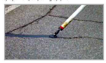
It can also be used to fill and over band the whole cracked area in combination with fine sand. A blanket cover is provided in such aphalt area having multiple cracks
